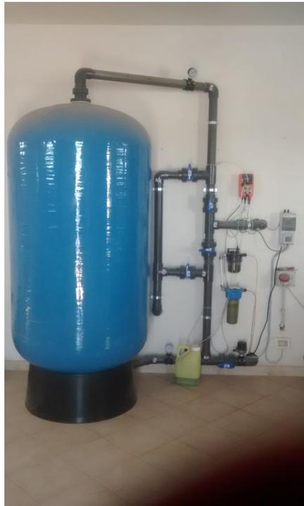
A module for correction of bad irrigation water
